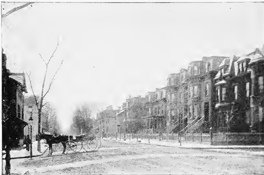
LIBERTY STREET—LOOKING SOUTH FROM CAMPBELL STREET.
